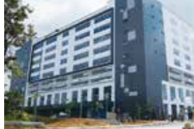
Malaysia Gapura project
