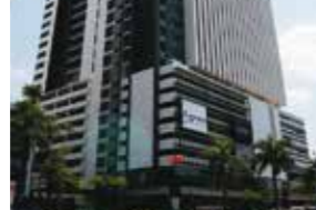
Malaysia Plaza 33 Office Block A
