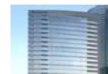
Heating & Ventilation A/C Company Headquarters
