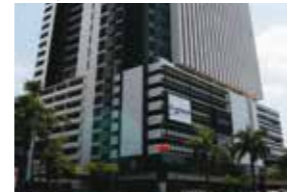
Malaysia Plaza 33 Office Block A
