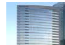
Heating & Ventilation A/C Company Headquarters
