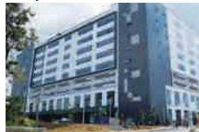
Malaysia Gaprana project
