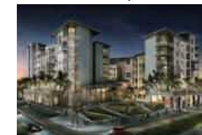
Panama Mosaic Building PANAMA PACIFICO
