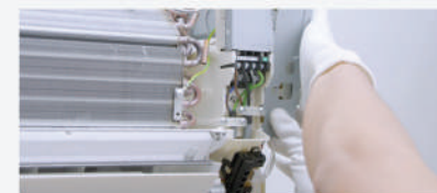
Remove control board cover.
