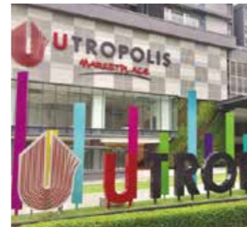
Paramount Utropolis / Malaysia - Installed in 2017
