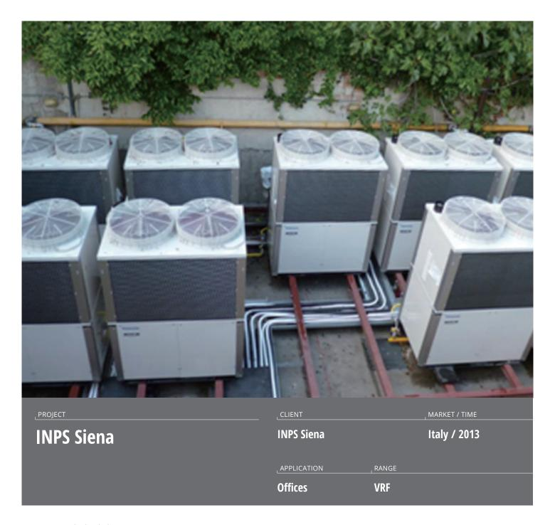
System: GHP + hydraulic kit Installation capacity: 822 kW installation Year: 2013
