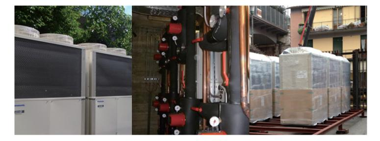
units. Each hydraulic kit controls a pump to move the water in the existing plant. The choice of this solution was determined by the following benefits: best economical tender, high performance in heating and cooling in severe weather conditions, powerful cooling/heating of the rooms, quite mode of the outdoor units, flexibility of installation.
