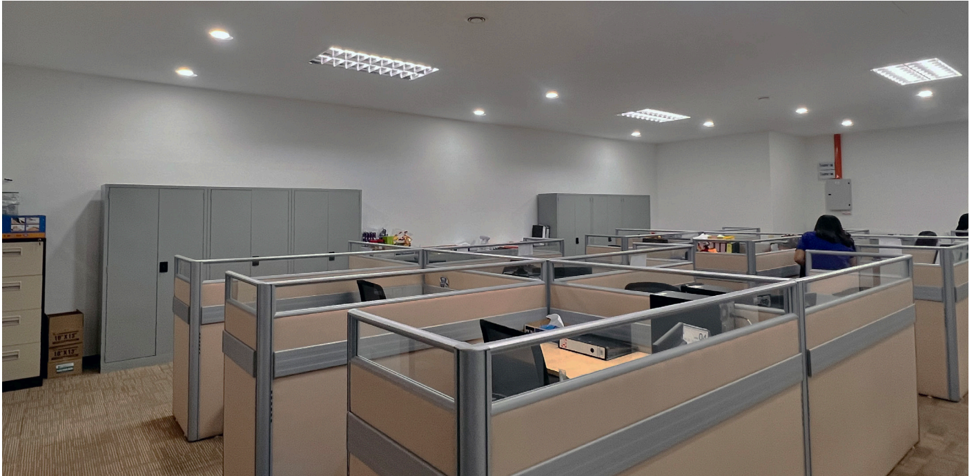
Neat installation of air-e nanoe™ X generator.
