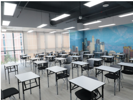
air-e nanoe™ X generator installed in one of the classrooms.
