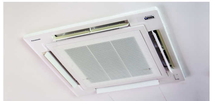
Cassette air conditioner equipped with nanoe™ X.
